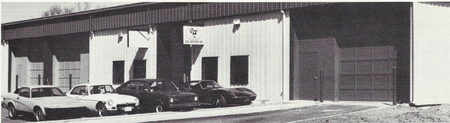
Group 44's new facility, front view. A Corvette seems to have crept in with the TR7, MGB/GT and Marina.
